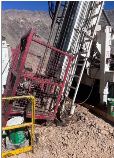
Figure 12.2: Drill Hole CMV-012b, Drilling
